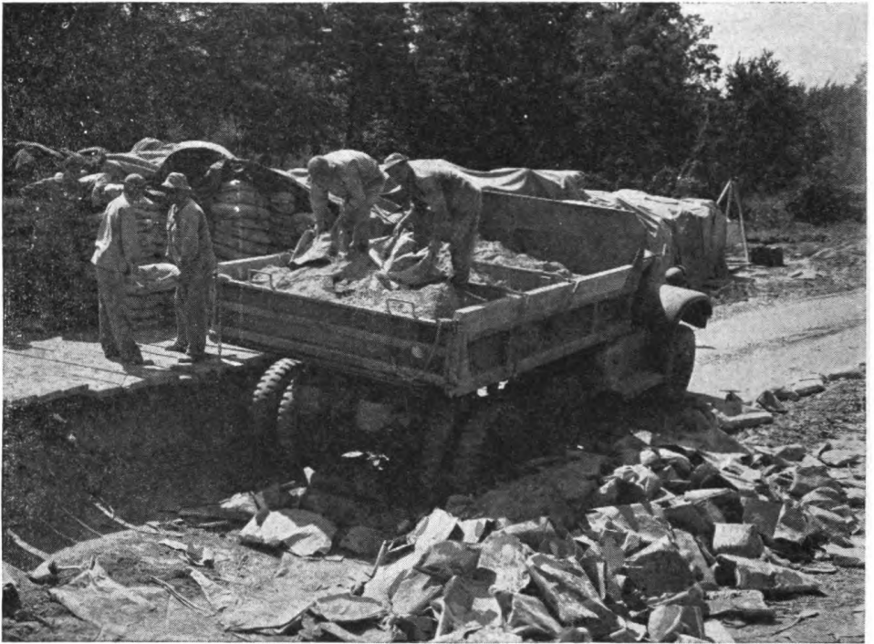
Figure 122. Adding cement at cement-loading point.
